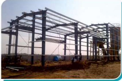
Processing Plant (PEB) at Panchmahal, Gujarat
