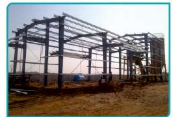
Processing Plant (PEB), Panchmahal, Gujarat
