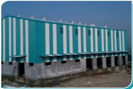
Pulse Mill, Dahod
