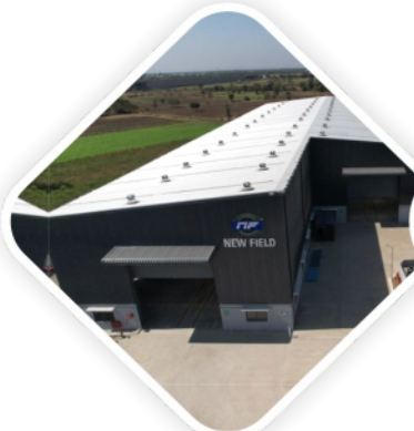
Engineering Unit measuring 42,000 sq ft at Gujarat
