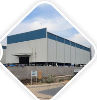
Engineering Unit measuring 10,000 sq ft at Gujarat
