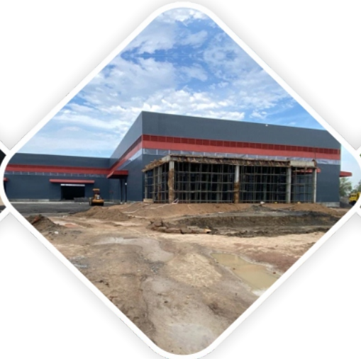
Engineering Unit measuring 66,000 sq ft at Gujarat
