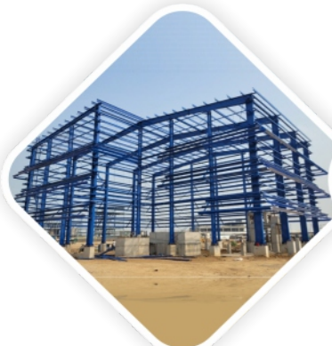
Chemical processing Unit measuring 7,000 sq ft at Gujarat
