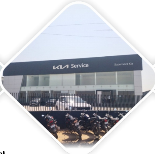
Showroom measuring 35,000 sq ft at Gujarat
