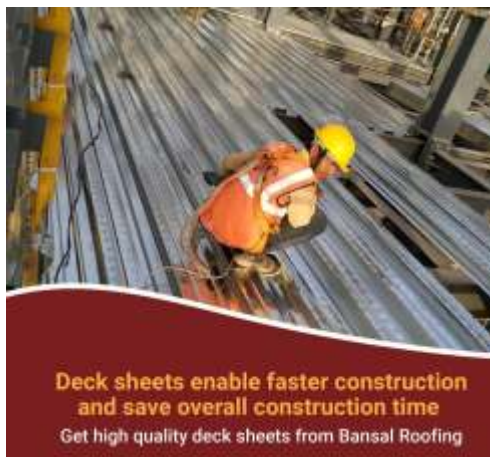
Installation of Deck Sheet
