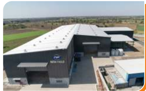
NEW FIELD ENGINEERING SAMLAYA
